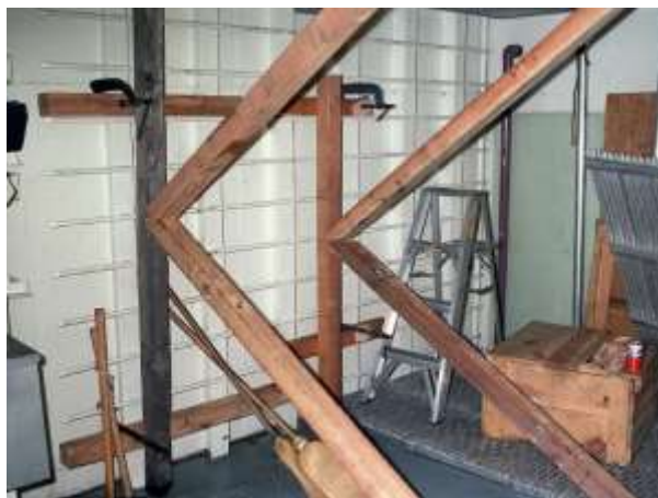
The crew fought flooding by emplacing K-type shoring, as well as using tool boxes and even their uniforms to stem the water pouring in.
