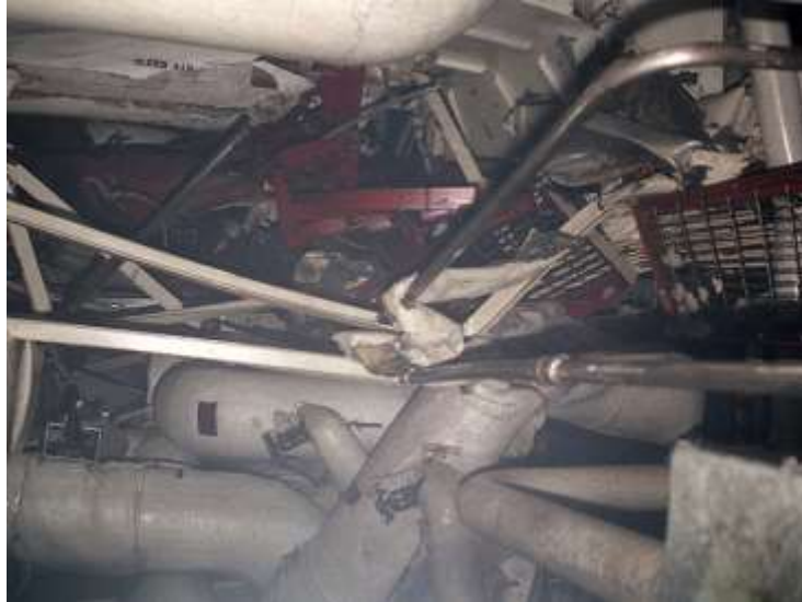
The blast tore through the ship's hull and bulkheads, completely flooding two main engine rooms
